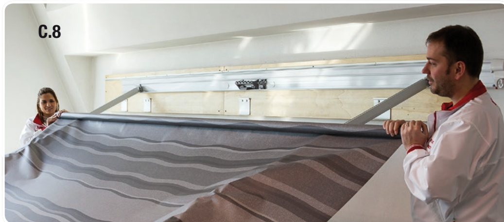
C.8 • Remove the roller tube from the right end cap and roll up the fabric.
